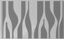
EXTERNAL FACADE PATTERN
